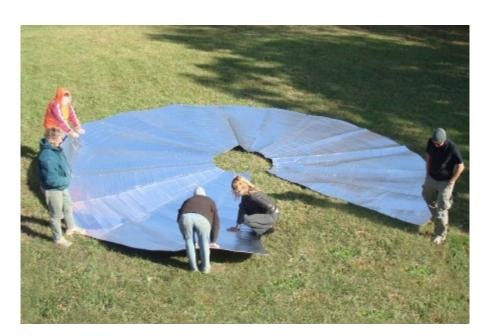
All roof insulation wedges are taped together for last seam (there will be a gap).
