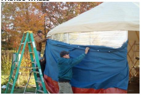
Hanging fabric wall with hanks to 1/8" cable in roof valance.
