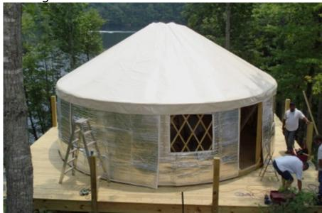
Wall insulation is installed. It should cover the front of the door frame(s), not just butting to it.
