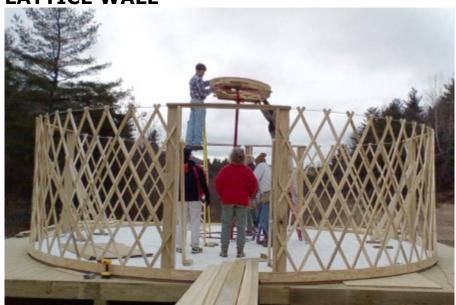
Lattice wall is level and attached to exterior side of "wings" on door frame. Tension cable is in place. Ring is elevated to proper height on lifter and ready to begin installing rafters.
