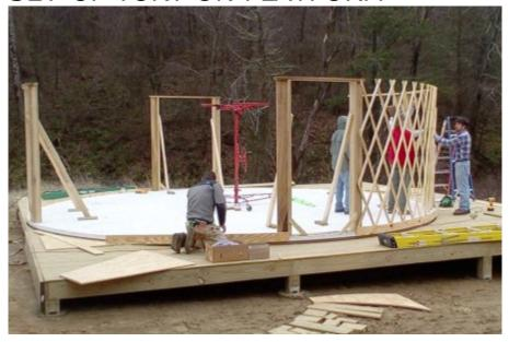
Door frames are set and plumb. Plywood band is being installed around bottom perimeter. Lattice wall is attached to exterior side of "wings" on door frame.
