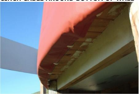
Bottom cable installed and tightened with turnbuckle.
