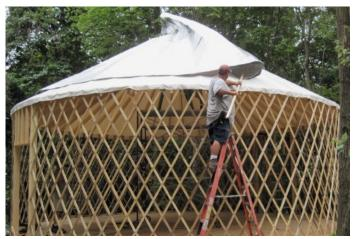
Cotton roof liner is installed. Notice the liner is hanging evenly around the top of the wall. The foil insulation layer is being unfolded with the help of the push stick.
