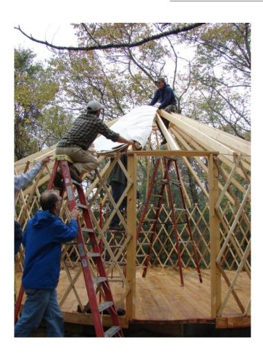
Cotton roof liner for roof insulation has been pulled up from outside the rafters and is ready to be unfolded.
