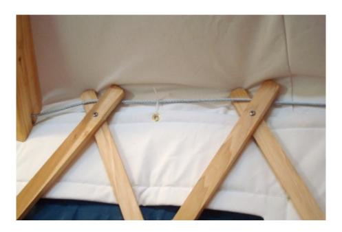
Wall insulation is hanging on 1/4" tension cable ties outside of the lattice.
